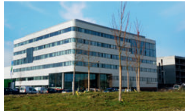
Logistics Cluster – 1st phase of construction
