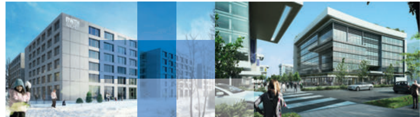
Production Engineering Cluster – 1st phase of construction
